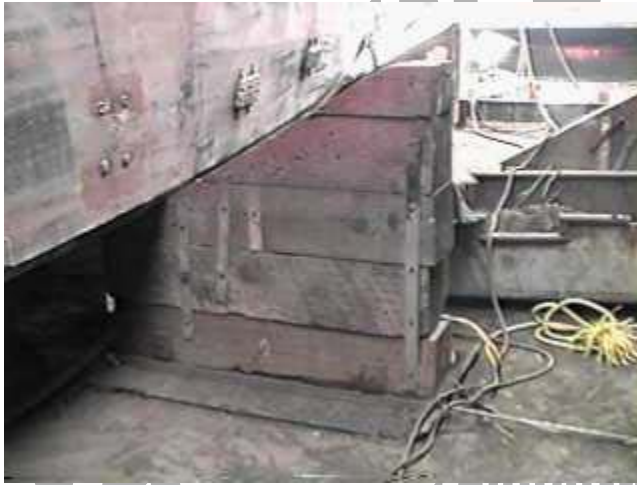
Bilge blocks supporting a vessel on a drydock.
