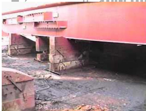
More bilge blocks.
